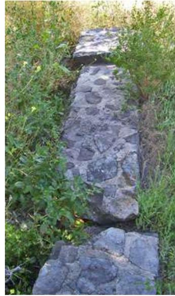
what is original and what is not. The only part of the right wall still awaiting repair is the very end, shown here. As can be seen, about 7 feet of the wall has broken away and is slowly sliding down the hill, toward the lake. What we have to do is uncover the base and lever the
