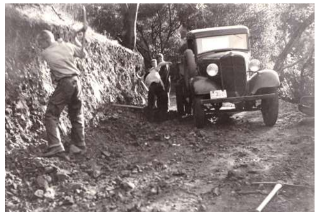
Road work, NE side of Dam, 1934
